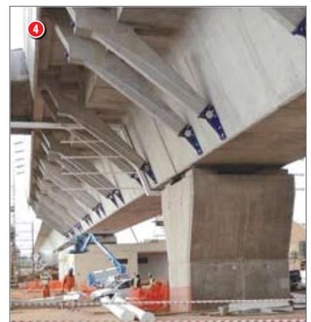
The standardisation of the pier head and standard 4 000 mm lifts allowed reinforcement cages to be prefabricated. This was advantageous considering the tight construction programme.
