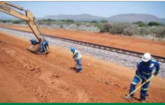
The Postmasburg link line under construction
