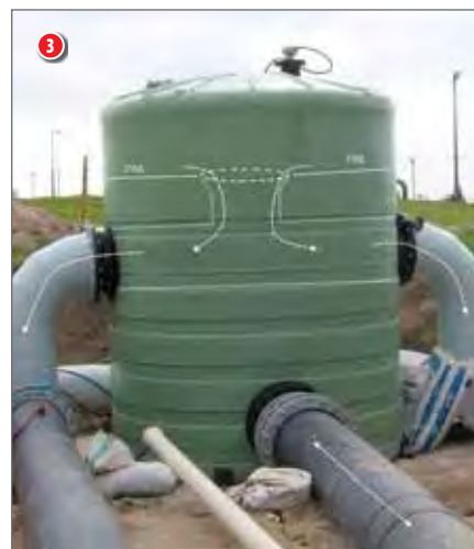
3 Photo 3: The BPS Famsys HDPE surge tank (before excavation backfill) c/w 450 NB HDPE inflow/outflow (surge) pipe and 400 NB GRP overflow / pressure relief pipework – normally dry (no signal from flow detector), but able to carry up to 0,5 cumec feed from internal 600 mm ND (variable elevation setting) drop-inlet spillway
