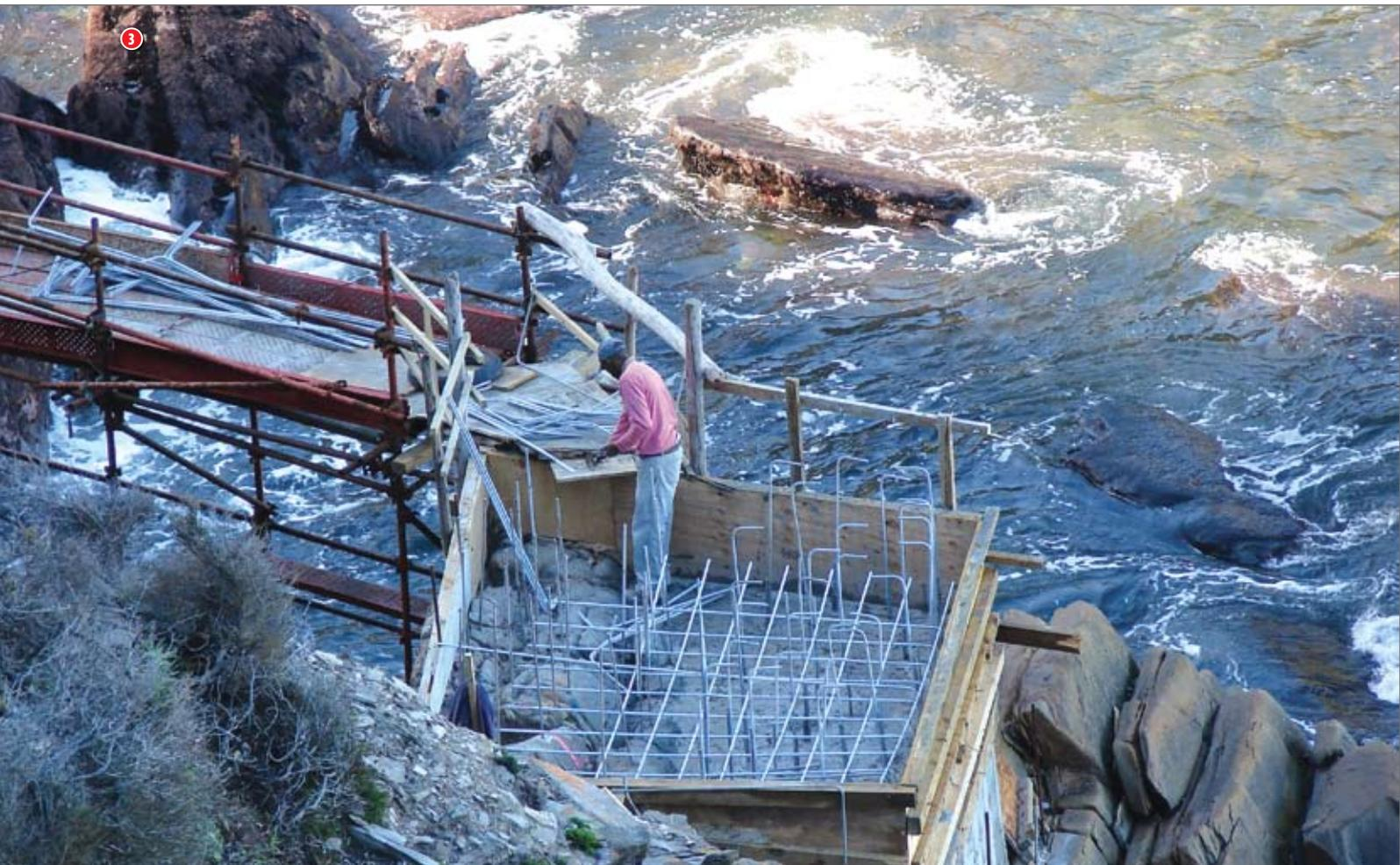
Concrete aggregates and cement were carried in, in 30 kg loads and stored in weatherproof containers at the easternmost (farthest) pier position. Concrete was mixed with a small mixer which likewise had to be partially dismantled and carried in. Water was obtained by a gravity siphon from the perennial stream near the start of the walkway, also 1 km from the site, and regulated by a simple garden tap at the outlet.
