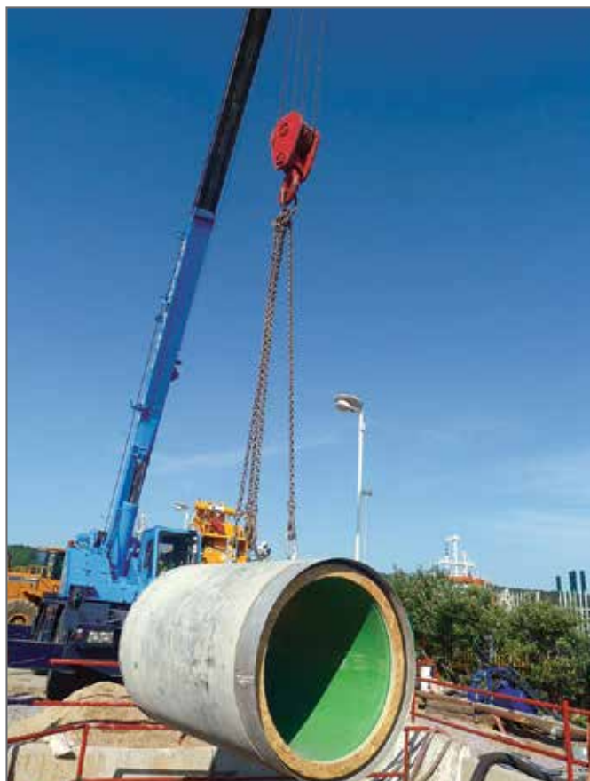
Each pipe was lowered into the jacking pit via a crane and inserted into the collar of the previously inserted pipe
