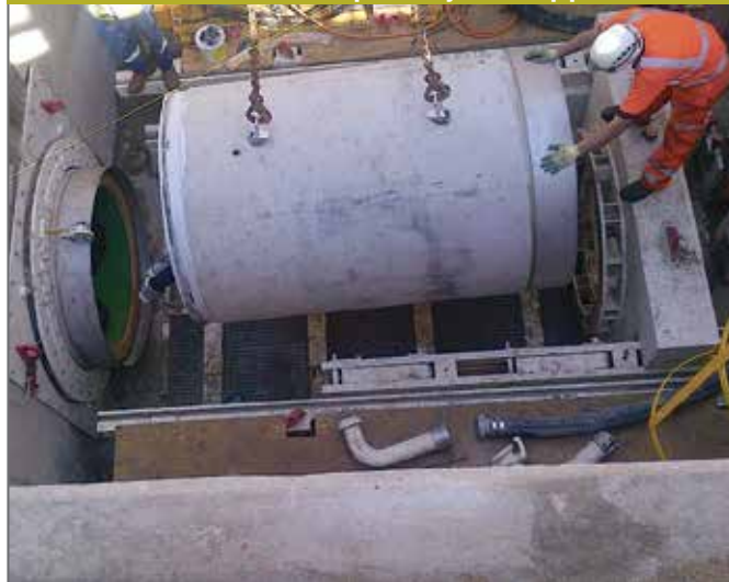
Each pipe was lowered into the jacking pit via a crane and inserted into the collar of the previously inserted pipe
