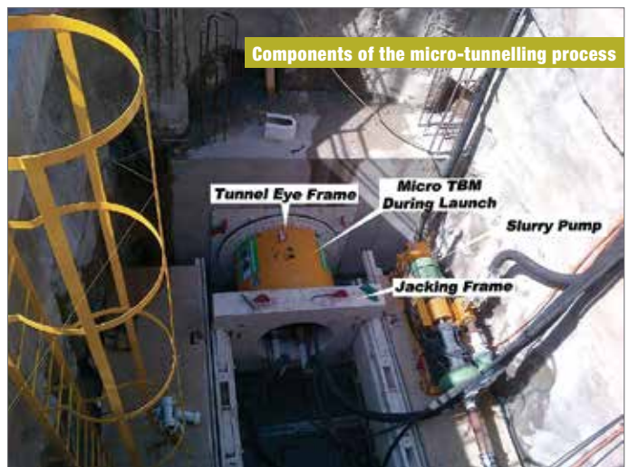
The micro-tunnel boring machine
