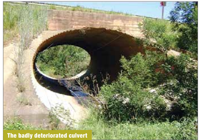
The badly deteriorated culvert
