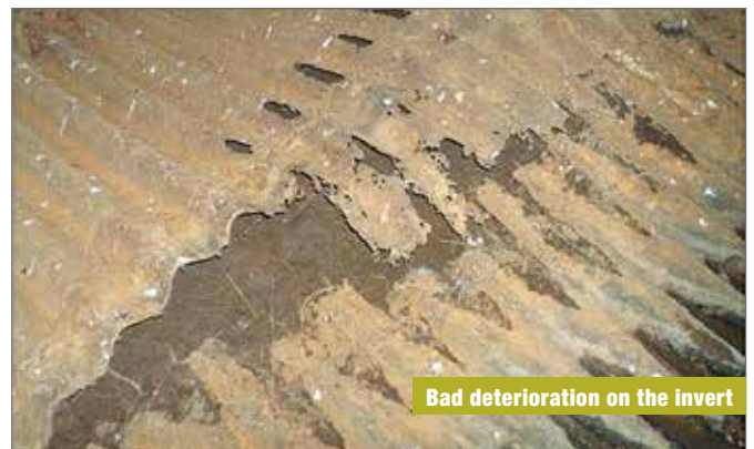
The badly deteriorated culvert
