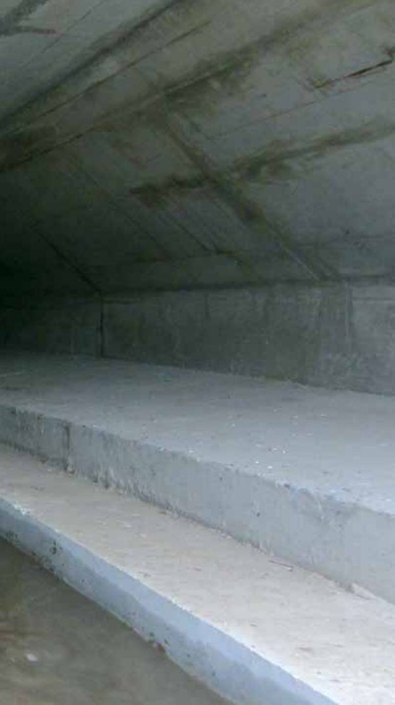
The badly deteriorated culvert
