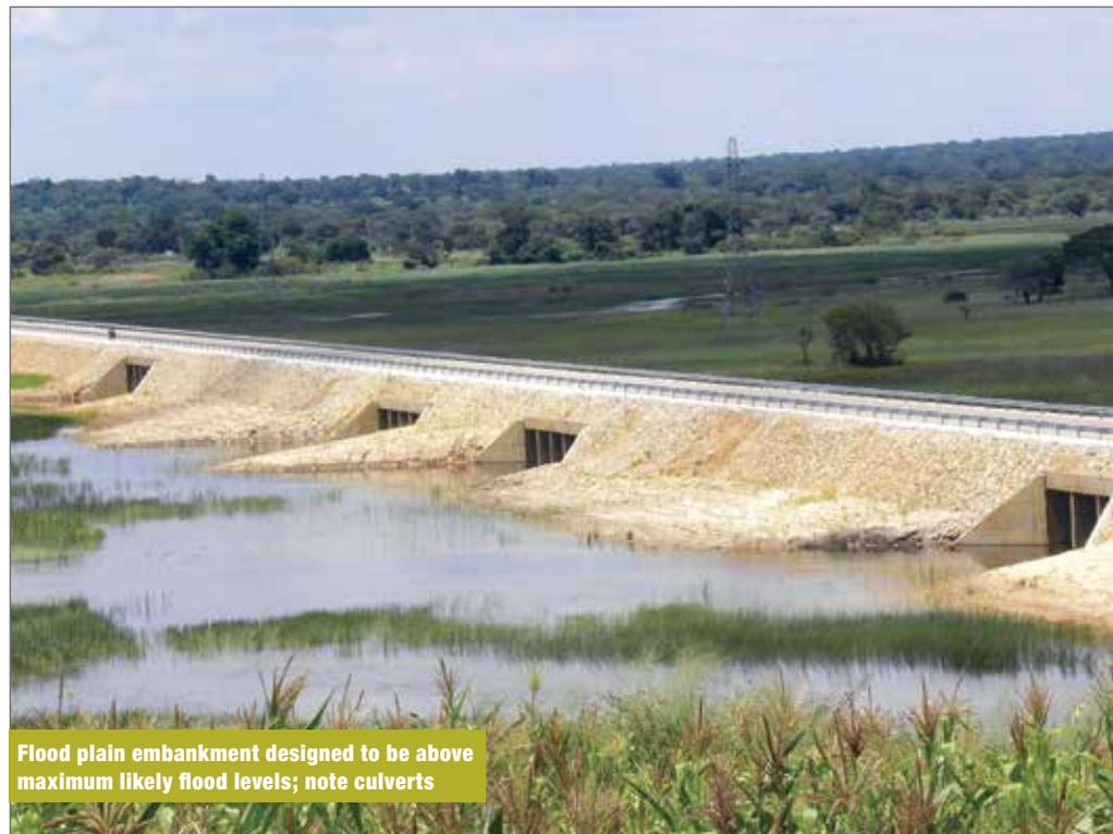
Flood plain embankment designed to be above maximum likely flood levels; note culverts
