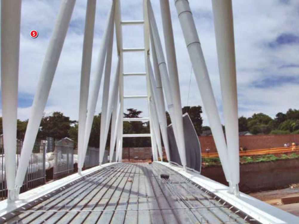
5 Leaning arch members and tapered cross bracing members
