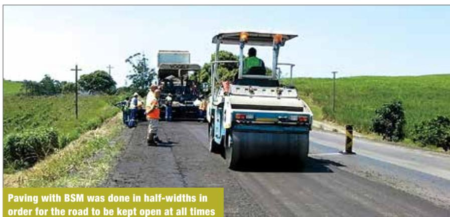
Paving with BSM was done in half-widths in order for the road to be kept open at all times
