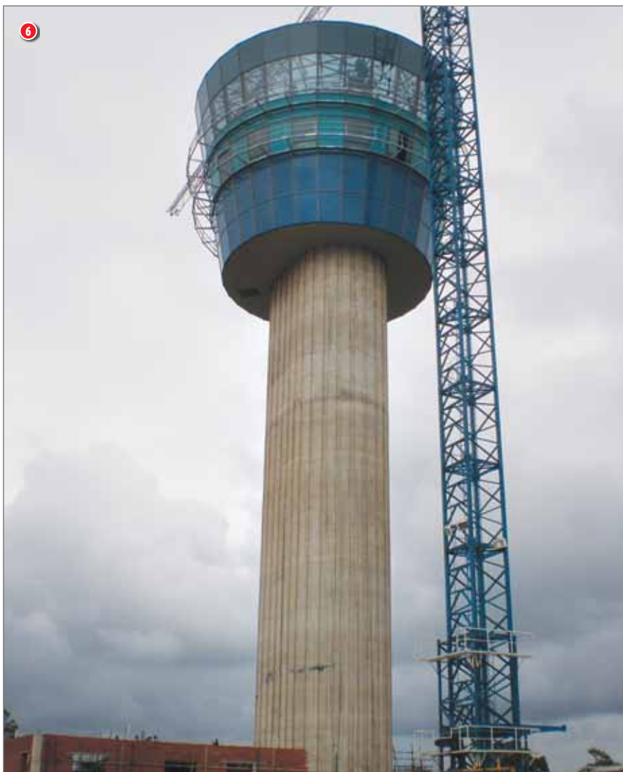
6 Control tower cab being erected
