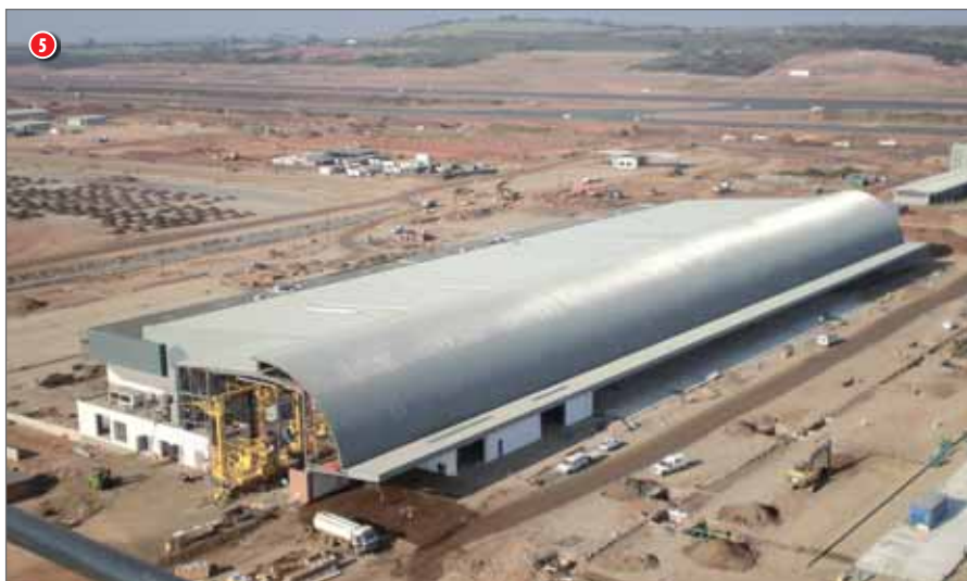
5 Completed cargo handling hall
