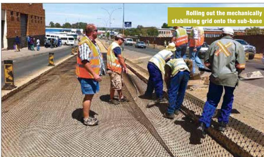
Rolling out the mechanically stabilising grid onto the sub-base
