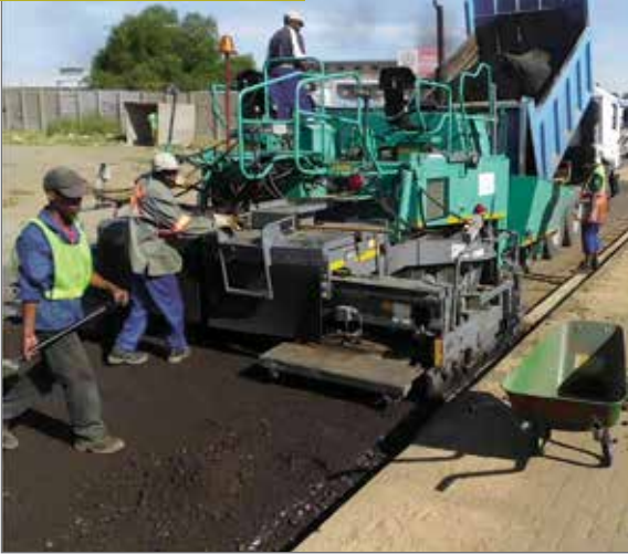
Asphalt paver working on top of the stabilising grid
