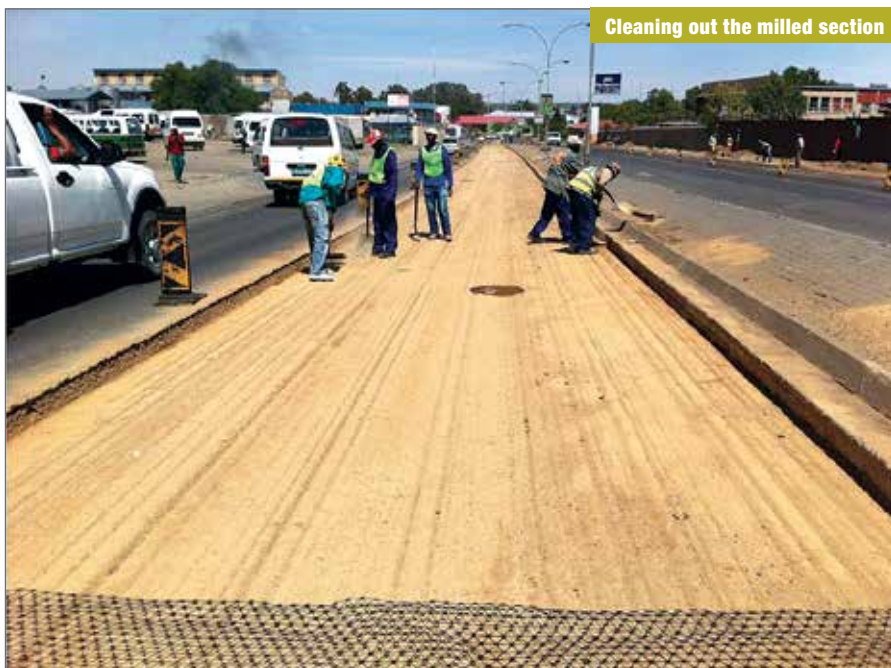
Rolling out the mechanically stabilising grid onto the sub-base
