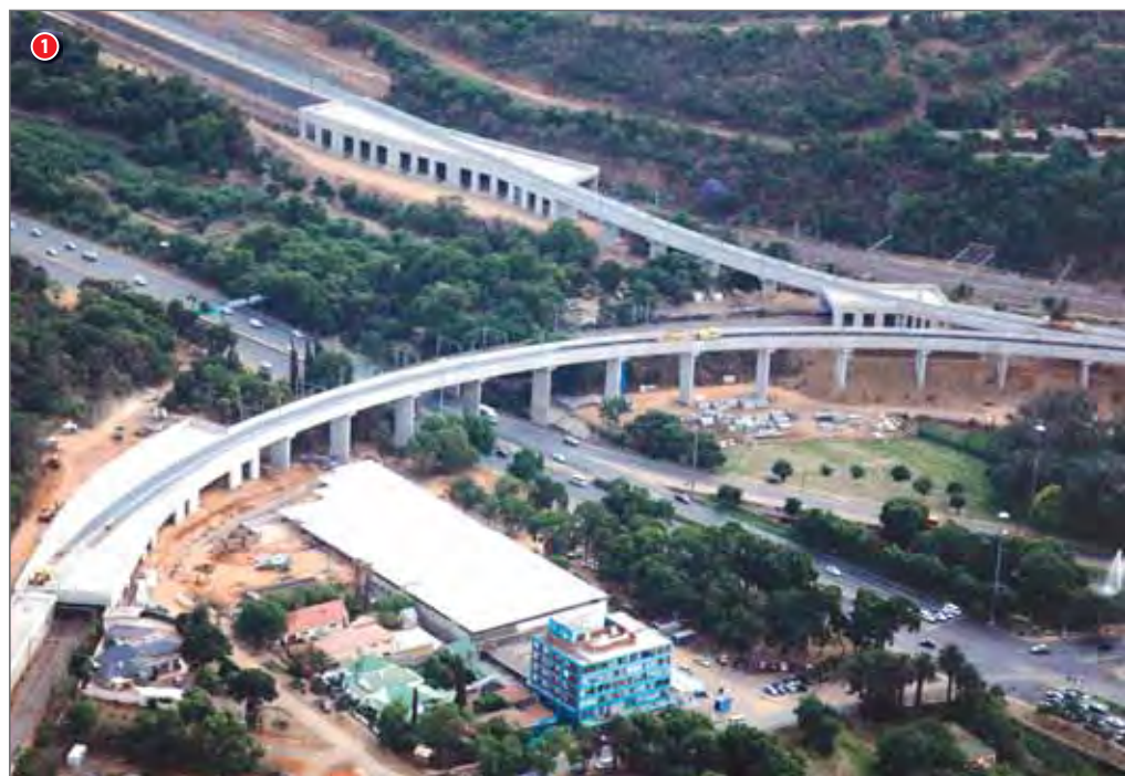
1 Gautrain flyovers and viaducts in Pretoria
