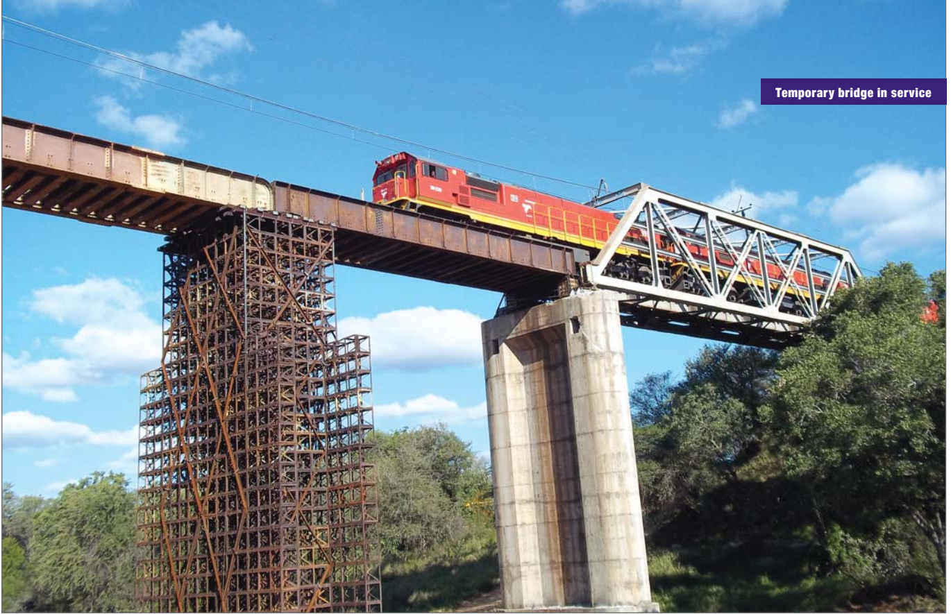
Construction of the new deck
