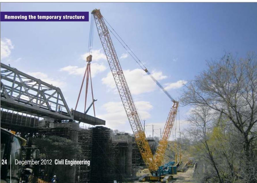
approximately 16.7 m long and space frame steel cribs fabricated from 50 x 50 angles.
